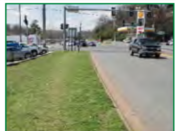
Commercial Road without Sidewalk
